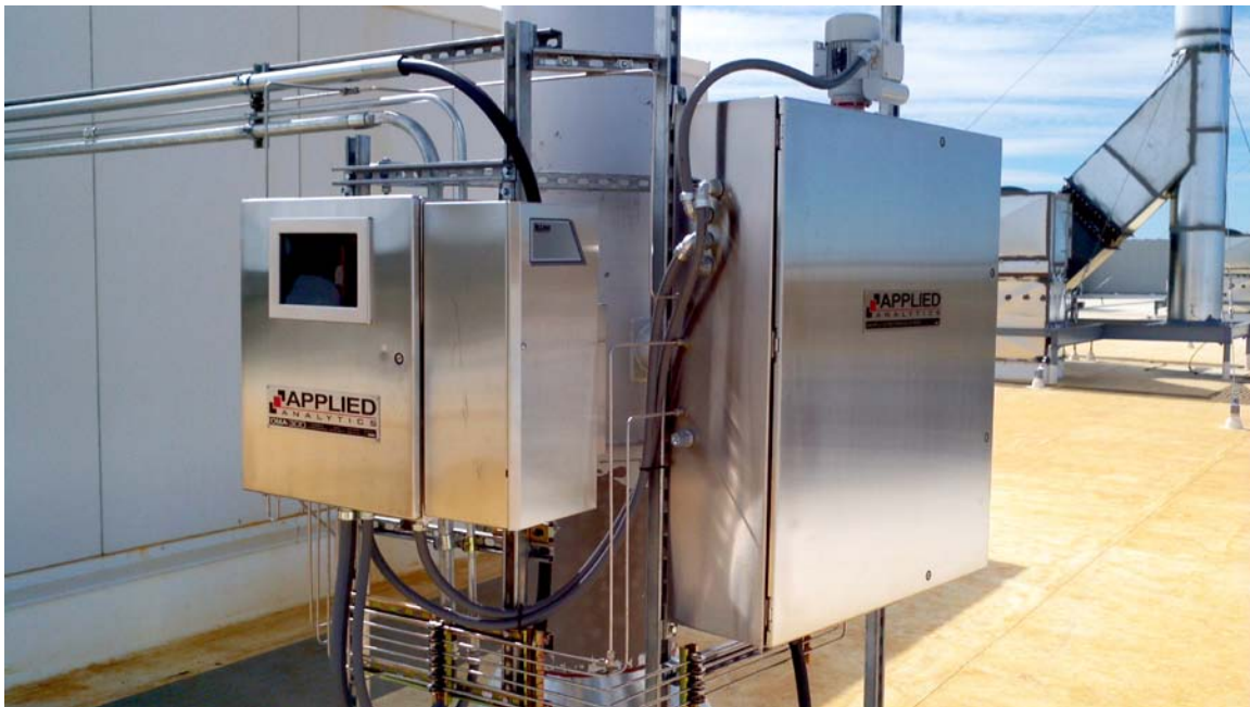
Example Installation: close-coupled OMA system analyzing flue gas at a manufacturing site.
